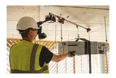
The weight of the unit being fitted is supported effortlessly by the hoist, making it easy for a single engineer to fix it into place. Indoor and outdoor (wind-rated) options available.
