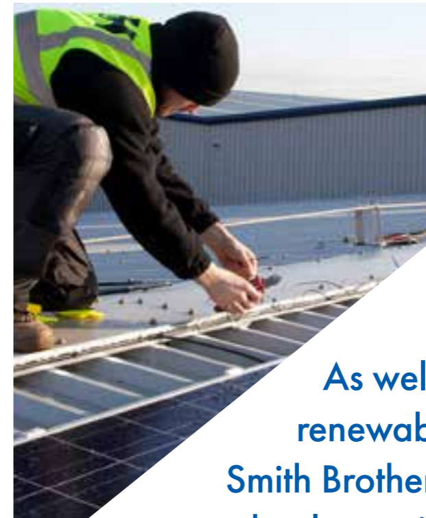
Leeds Solar Install
